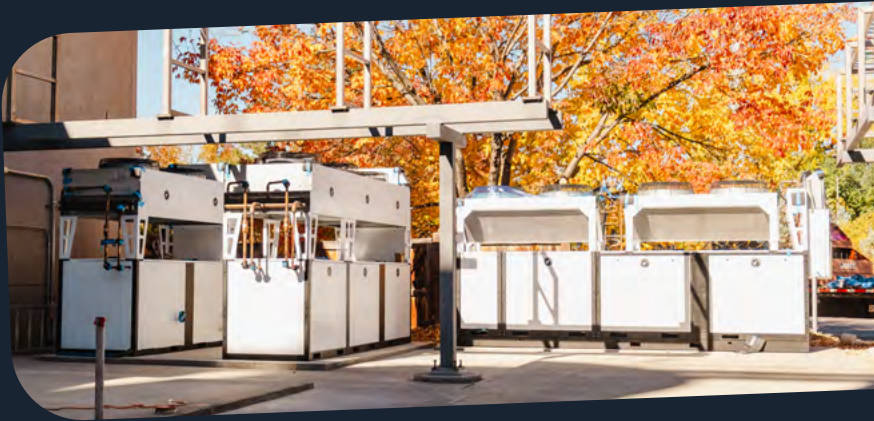
Installing the CO 2 Recovery System. The large blue container comprises our system for cleaning, compressing, and liquefying captured CO 2 , while the white units are chillers for liquefying CO 2 . The farthest right chiller unit is a groundbreaking unit developed in partnership with G&D Chillers. This innovative unit uses propane, a natural refrigerant with no ozone depleting potential, and global warming potential equivalent to CO 2 .
